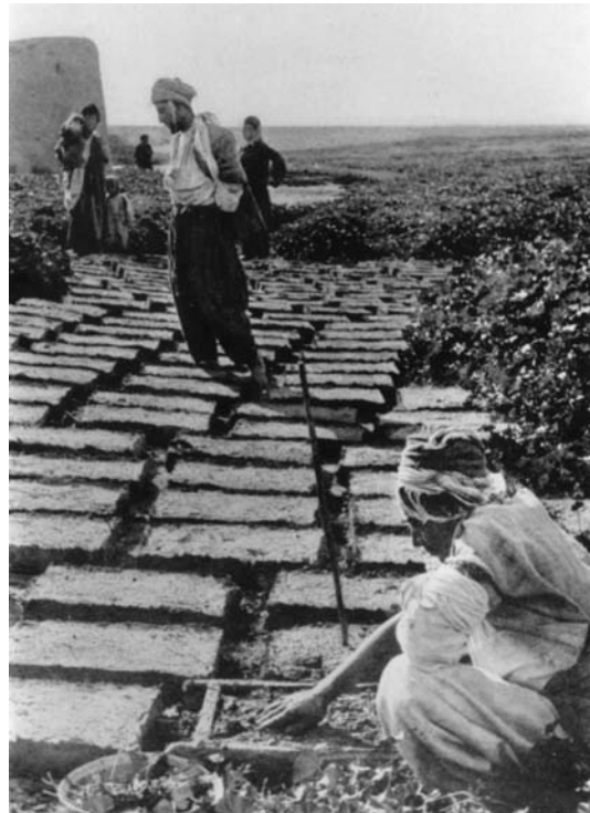
6.1 Making sun-dried brick near the bank of the Tigris River. (Rogers, A History of Babylonia and Assyria , 1915)
