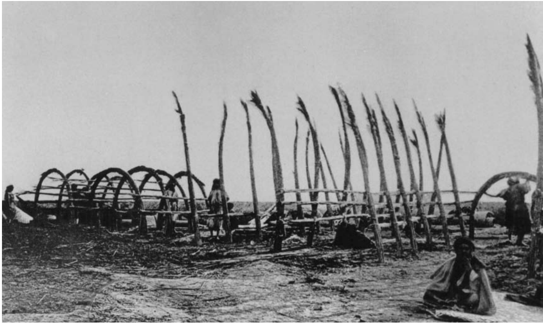
6.2 An early 20th-century view of reed houses being constructed in southern Iraq using age-old techniques and design. (Rogers, A History of Babylonia and Assyria , 1915)
