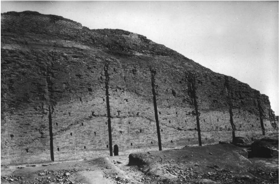
6.5 In this exterior view of the ziggurat at Ur, we can make out downspout channels and “weep holes” in the brick façade. These were designed to keep the interior of the structure dry. (University of Pennsylvania Museum)
